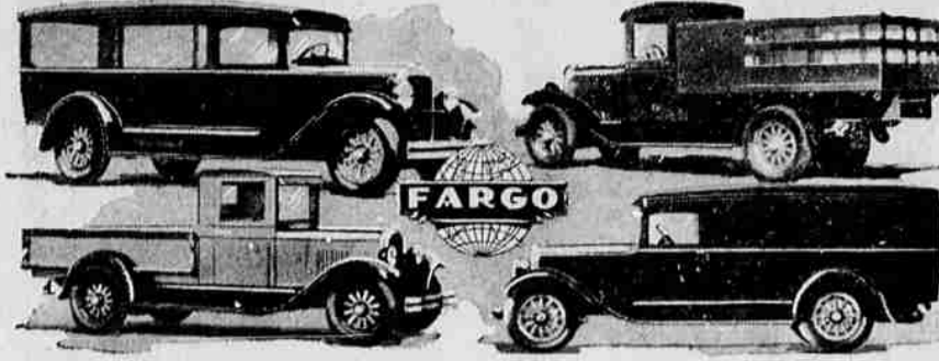
Here are four body styles of the "Freighter", new product of the Fargo Motor Corporation, truck division of Chrysler. The Freighter has a wheelbase of 133 inches and is powered by a 55 h. p. Chrysler six-cylinder engine. Fargo has been building 1/2 and 3/4 ton delivery equipment for eight months. The "Freighter" has just been added to the line.
