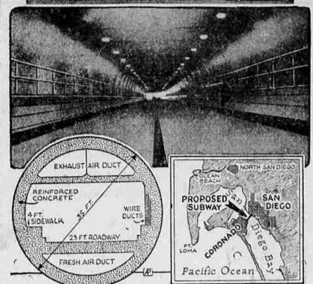
A tunnel such as the one above will connect San Diego and Coronado, Cal., under the waters of San Diego bay. The cross section (lower left) shows the type of construction, while the map at lower right shows the position of the two cities.
