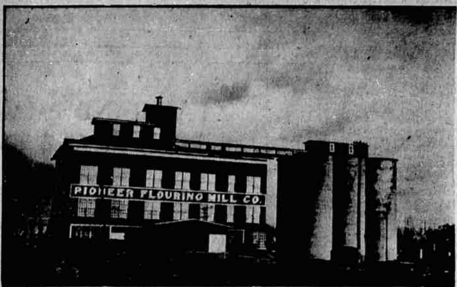
Here is an excellent picture of the Pioneer Flouring mill plant at Island City, where the headquarters of the company are located. The plant pictured above is one of a group of mills over Union county which handles a remarkable amount of locally grown wheat, grinding it into flours of various kinds. The company's markets international in scope.
