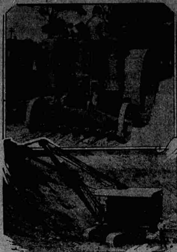
New road machinery is influenced by the trend in automotive machinery. The motor driven roller (above) fast is replacing the old time steam roller, while the new shovels mounted on caterpillar tractors do six times the work of their predecessors.
