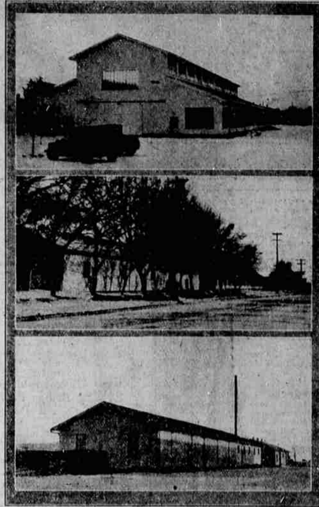
Here are three views of the equipment warehouses and shops erected at La Grande during 1928. The upper picture is of the main building, in which the machine shops, etc., are located. In the center is a view along East Adams avenue. The bottom picture shows one of the warehouse buildings. A sixth structure is now being erected at the plant.
