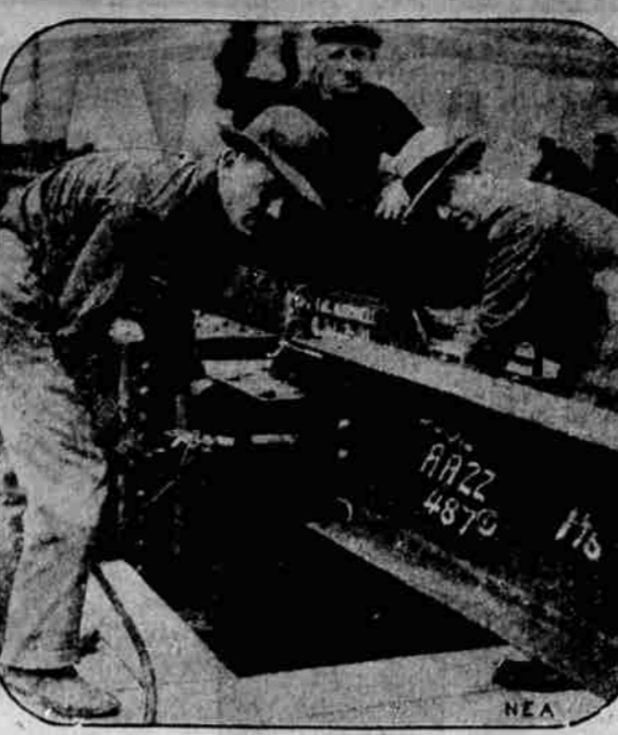
The steel superstructure of the world's biggest business building, the Merchandise Mart in Chicago, has begun to rise above the Chicago river at Wells street. James Simpson Jr., son of the millionaire president of Marshall Field & Co., is shown driving the first rivet in the steel framework. The building will house 2000 prominent manufacturers, wholesalers and importers. Young Simpson has been helping with the construction work. On the right is shown C. A. Welles, general manager of the Merchandise Mart.
