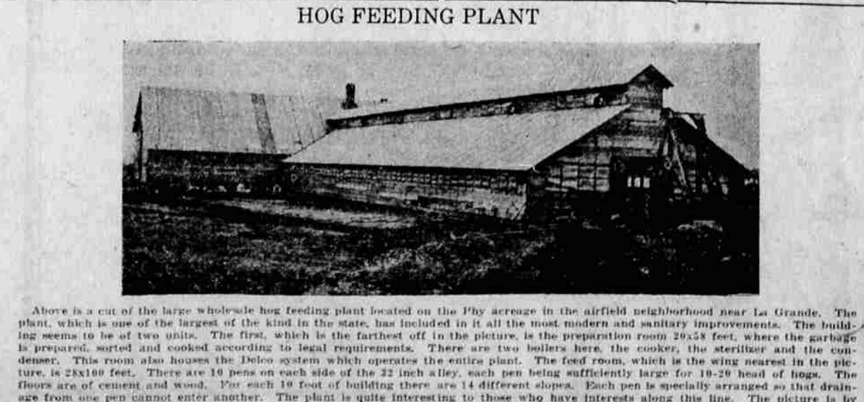
Above is a cut of the large wholesale hog feeding plant located on the Phy acreage in the airfield neighborhood near La Grande. The plant, which is one of the largest of the kind in the state, has included in it all the most modern and sanitary improvements. The building seems to be of two units. The first, which is the farthest off in the picture, is the preparation room 20x8 feet, where the garbage is prepared, sorted and cooked according to legal requirements. There are two boilers here, the cooker, the sterilizer and the condenser. This room also houses the DeLoe system which operates the entire plant. The feed room, which is the wing nearest in the picture, is 28x100 feet. There are 10 pens on each side of the 32 inch alley, each pen being sufficiently large for 10-20 head of hogs. The floors are of cement and wood. For each 10 foot of building there are 14 different slopes. Each pen is specially arranged so that drainage from one pen cannot enter another. The plant is quite interesting to those who have interests along this line. The picture is by Mae Stearns.
