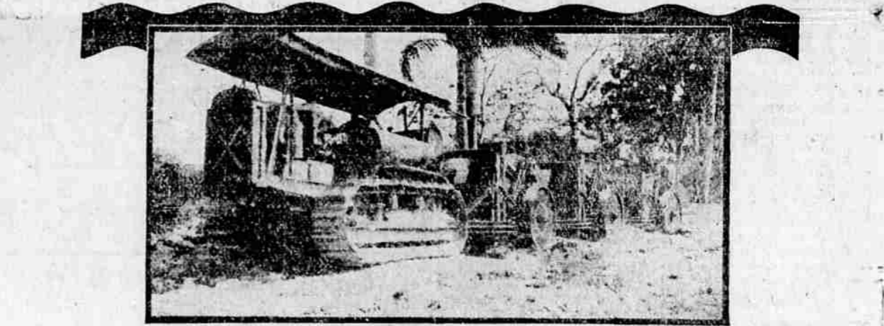
A "Sixty" Moving Earth on a Road-Building Job in Cuba
