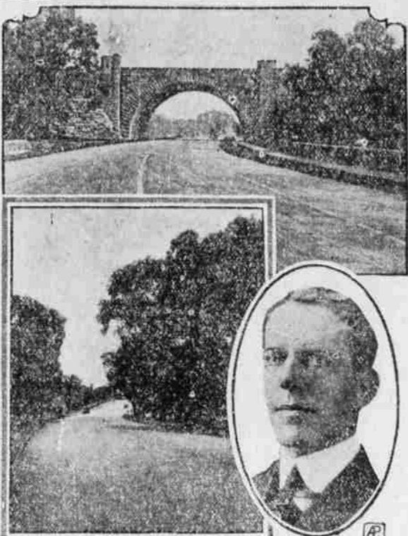
The Hutchinson River Parkway (lower left) in Westchester county, New York, providing a four-lane highway for passenger automobiles, has solved a suburban traffic problem common to American cities by insuring a steady flow of traffic at 35 miles an hour. Intersecting roads and railways are sent across the parkway on arched bridges (above). V. Everett Macy, president of the Westchester County Park Commission (lower right), led the movement for construction of the roadway.
