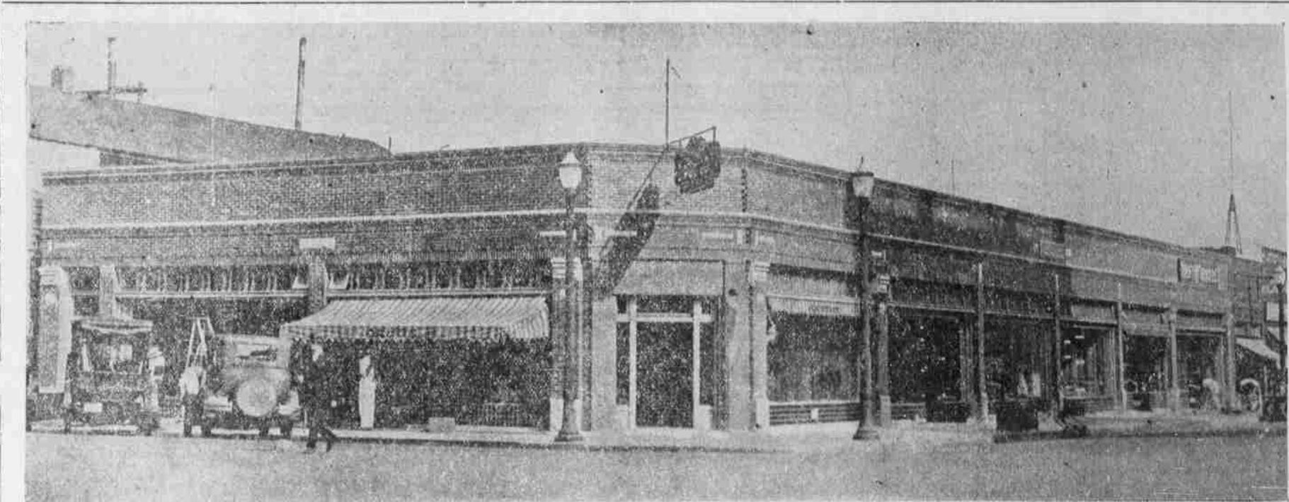
This is a view of the new Grace building, on the corner of Adams and Fir, taken from in front of the M. J. Goss company location. It shows the corner room which is being occupied by the Moon Drug company and the additional rooms fronting on Adams. Next to the Moon store is the 66-foot front of the new Stevens-Van Engelen department store. The next store is occupied by the Grace Harness shop operated by the owner of the building, Mrs. Grace Snyder. The last store in the new building is the new Thrift Grocers store, which is the second cash store established in La Grande by the La Grande Grocery company. The Thrift store extends all the way back to the alley while the other stores have a depth of 60 feet. W. Vedder was the general contractor and Charles E. Miller the architect.
