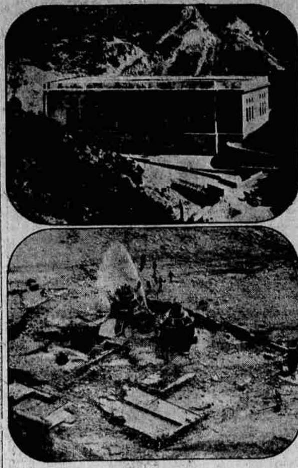
Here is graphically pictured destruction wrought by the wall of water that swept through the San Francisco canyon near Los Angeles after the St. Francis Dam broke. The half-million dollar power plant at the foot of the canyon, the first building to be struck by the flood forces, is pictured before and after the disaster that wiped out the ponderous concrete structure. Only two of the great turbines and the foundations of the building are visible.
