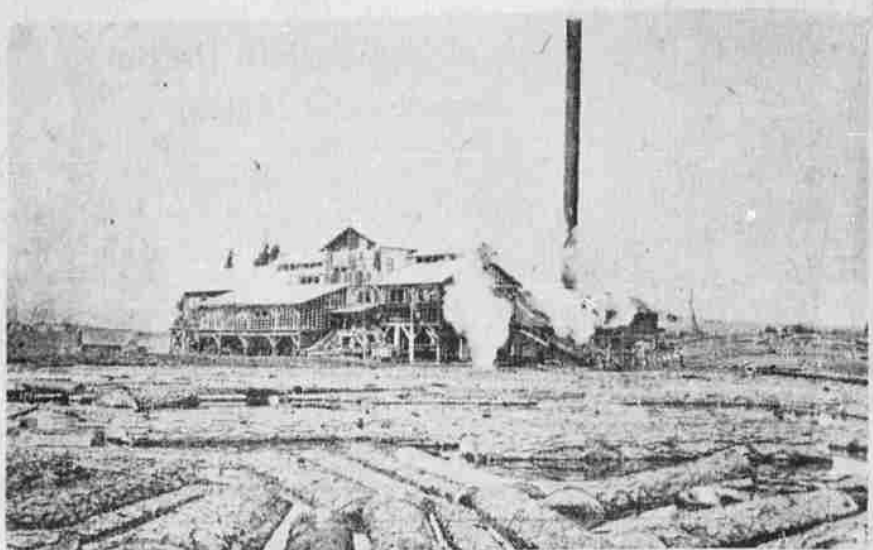
The mill of the Grande Ronde Lumber company recently erected at Pandosa, lying near the southern border line of the county. The view is the rear of the mill, taken across the log pond and looking toward the road. At the extreme left hand side may be seen a few of the cottages erected by the company for the mill employees.
