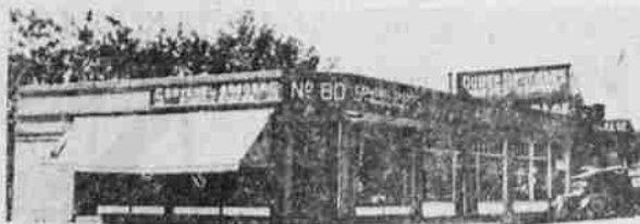
One of the latest blocks to be built up in La Grande is the above brick business block, which represents a part of the ever expanding business section. The building was erected last year by L. C. Smith, proprietor of Dodge Brothers garage which is adjoining the new Smith building. Scrivens Grocers No. 80 occupies the first store room in the building and the next is the Grist, Marshall beauty shop. The third store room is occupied by Green's Repair shop. The fourth store room is used by Mr. Smith as a show room for his Dodge cars.
