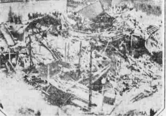
Above is the wreckage of a four-story Chicago department store that collapsed while an anniversary bargain sale was in progress. It was feared hundreds were killed, but rescuers reported there were no fatalities. The walls of the building were said to have been weakened by steam shovel excavations next door.
