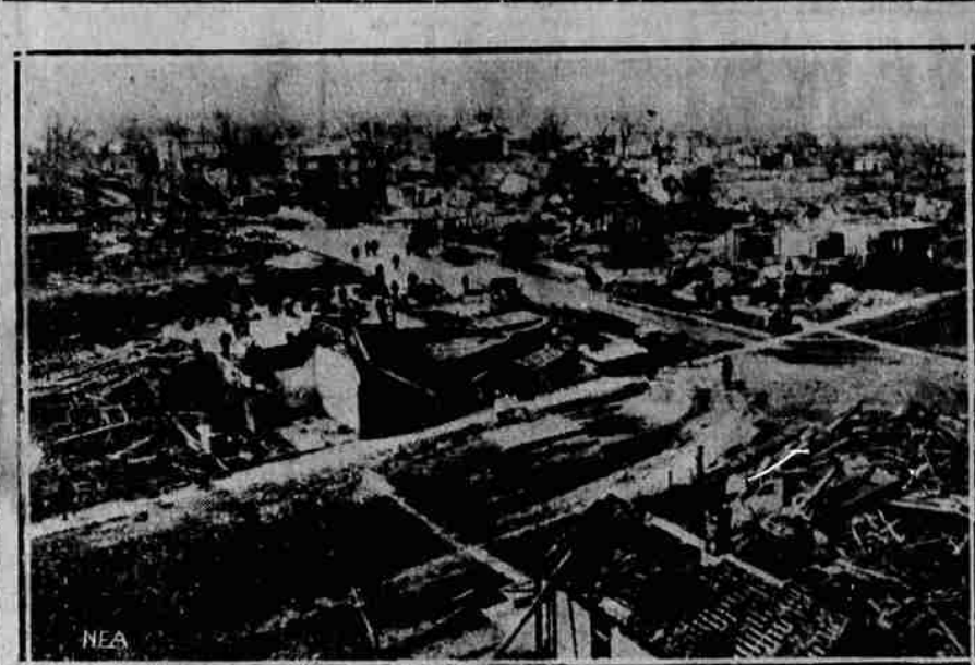
1927. NEA Service, Inc. Transmitted by telephoto. Photo Copyright. This remarkable telephoto picture shows the damage caused at Cornland, Ill., by a tornado that swept across the state, taking about 55 lives. Every building in the town was demolished or dam- aged, and people are shown seeking their belongings in the ruins. The picture was taken from the top of a badly damaged grain elevator.
