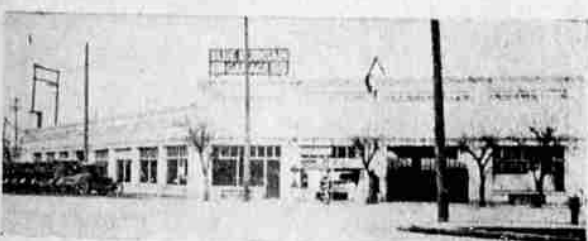
The Blue Mountain garage, located on the corner of Fourth street and Adams avenue and facing the latter, was erected a few years ago. The building was especially built for the use of Avery Harrison, Chevrolet distributor here, and affords him adequate space for his business.
