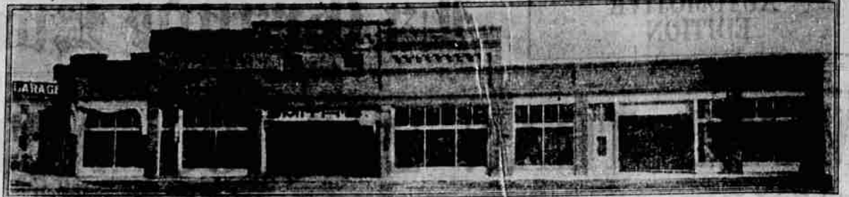
L. C. Smith, pioneer automobile dealer of Eastern Oregon, has a large amount of floor space available in this building. He recently built an addition and has a new show room. His garage is located at the corner of Fifth and Depot streets.
