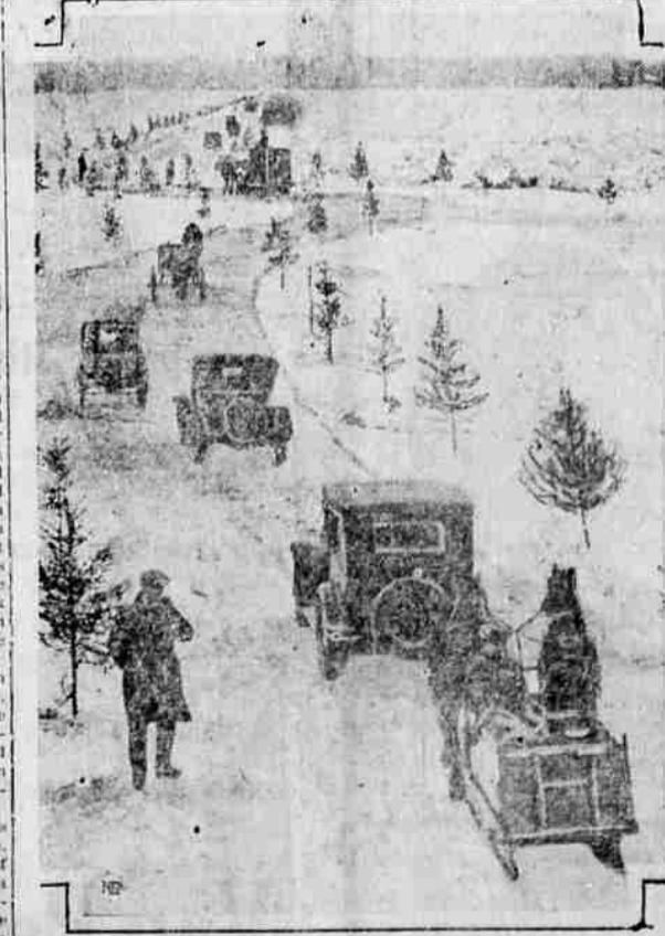
The famous Queen Victoria bridge over the St. Lawrence river at Montreal, Quebec province, is closed for repairs, but traffic isn't inconvenienced much. Motorists and such so right across the bridge—the river is traversed over safely. This photo shows the route, marked by rows of small trees (planted from nearby hills).
