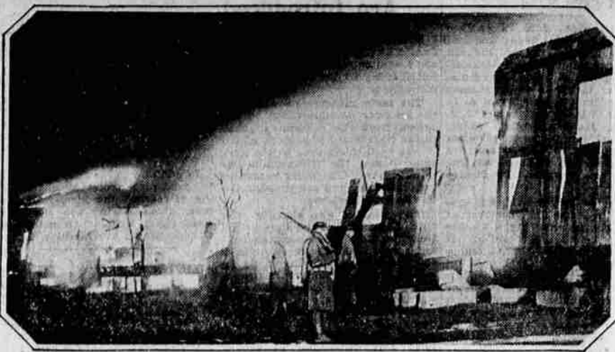
Doughboys, coast guards and firemen worked five hours to subdue flames which threatened the Second Army Corps headquarters at Governor's Island, New York, while destroying four old barracks buildings. A dozen men were slightly injured or overcome by smoke. The fire's damage was estimated at $100,000.
