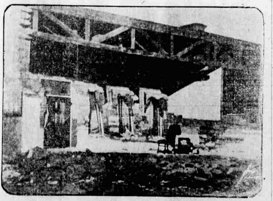
TELEPHOTO—Recurrent earth tremors did $2,500,000 damage in southern California and northern Mexico on New Year's day. There were no fatalities. In the lower Imperial Valley, the quake's hand was laid heaviest on Calexico. This view of the wreckage of the Pioneer Transfer company's U. S. bonded warehouse there was relayed by motorcycle to San Francisco, telephoted to New York and hurried to The Observer by NEA Service.
