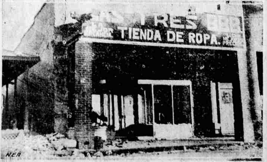
Pedestrians were imperiled by the falling bricks from walls like this, and there were many narrow escapes. Photo shows a damaged mercantile establishment in Mexico.
