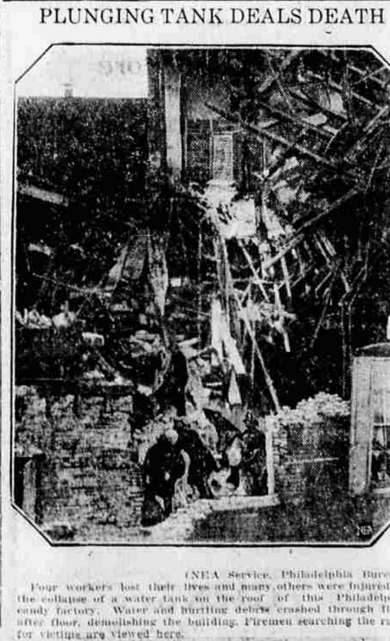
Four workers lost their lives and many others were injured by the collapse of a water tank on the roof of this Philadelphia candy factory.
