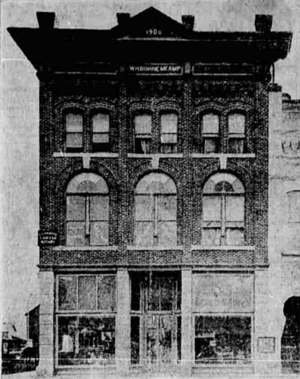
Above is a picture of the building W. H. Bohnenkamp erected in 1900, taken just after completion. The company occupies a part of this building now. The two upper stories were destroyed by fire several years ago and the building was remodeled, three upper floors replacing the original two.
