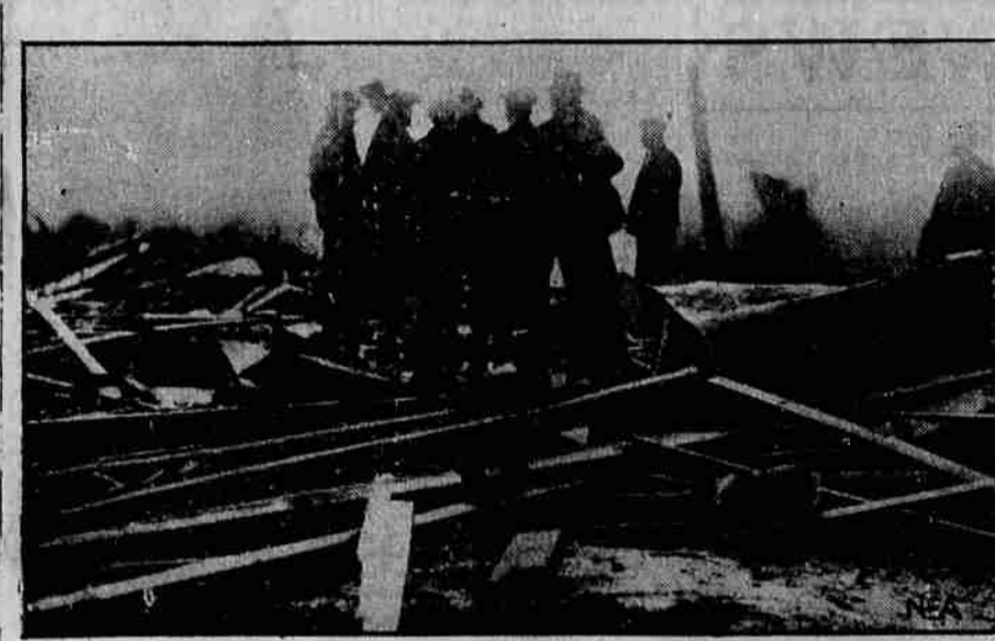
All that was left of the village school house at Ly Plata, Md., after a tornado struck it, killing 15 children, is pictured above. Unwarned of their peril, the school children were crushed by falling walls and hurdling timbers, or blown bodily through the wreckage, out over the grounds. A score were taken to hospitals, badly injured.
