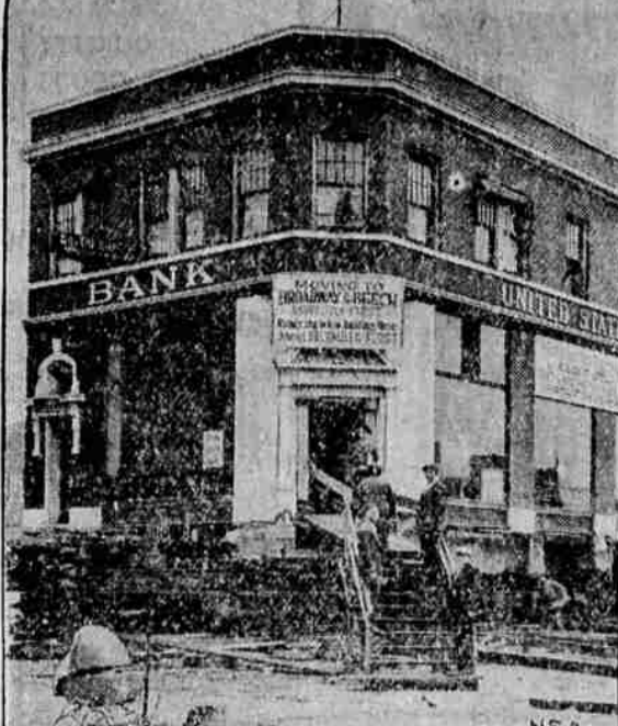
When the United States National Bank at East Chicago, Ind., started to build its new building, it had to move the old one to a vacant lot a block away. President Walter J. Riley insisted there must not be a minute's interruption of business. So throughout the ten days it took to move the bank, business was carried on as usual.
