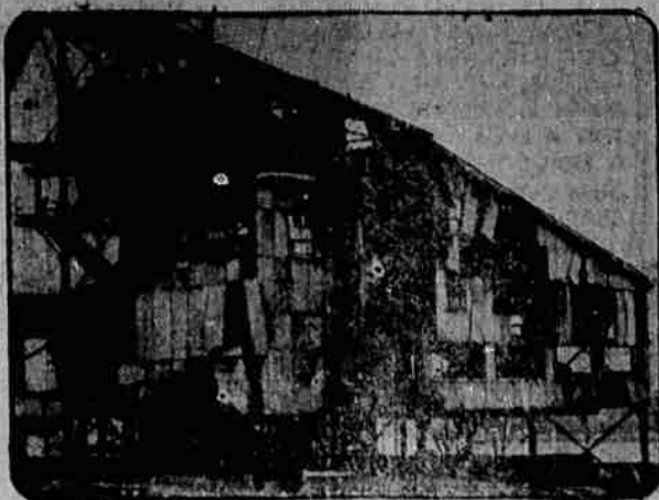
The main shaft of the Cleveland & Western Coal company's mine at Poughatan, O., was wrecked, one man was killed and twenty-two were injured by a coal dust explosion—but 600 men in the mine escaped unhurt because rock dust had been sprinkled on the floor and walls. Photo shows the wrecked mine tipples at the top of the shaft.
