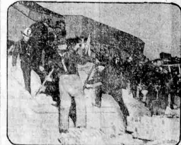
Five men were killed and four others hurt when a one-story San Francisco factory building collapsed due to undermining of the walls by a contracting firm that was excavating for a new building next door. Photo shows fire men working by lamp light in the search for more victims.
