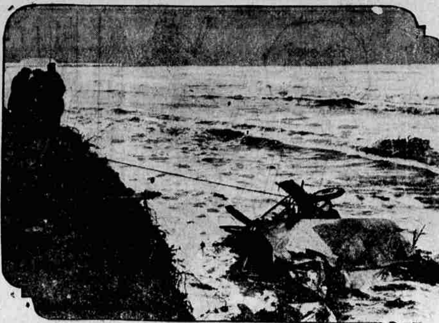
Considerable damage, largely to the local pride of the citizens, was done when a rain-storm swept the coast of Florida. This picture shows a Curtis seaplane wrecked by high seas and driving rain off Daytona Beach.
