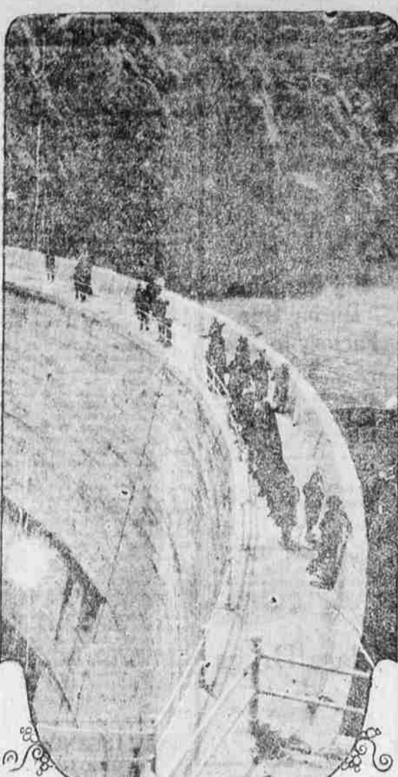
MOST REMARKABLE PIECE OF ENGINEERING among the many that have made the desert to flower in the west, Shoshone Dam on the Yellowstone River in the national park. Each year thousands of tourists pass through the park, and nearly all of them visit this dam. The walkway along the top of the dam makes an ideal promenade for visitors.
