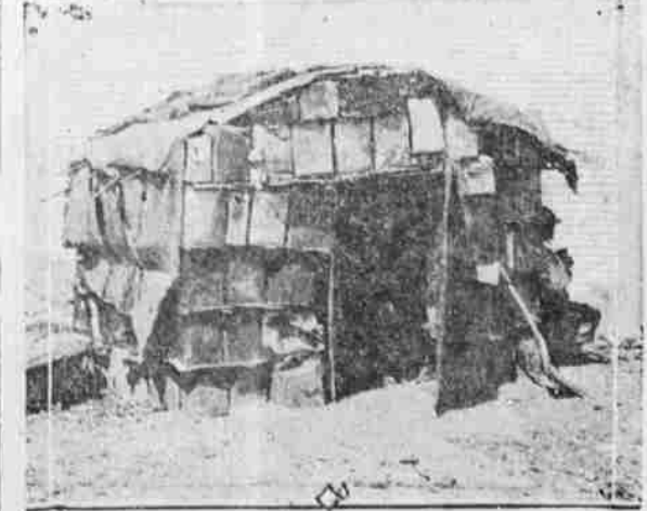
KEROSENE OIL CANS are preferred by prospectors to stone in building cabins down in Patagonia. The cans are filled with clay and wired together.
