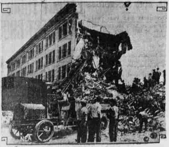
Santa Barbara is hard at work repairing the devastation wrought by her earthquake. This picture shows workmen busy on the ruins of the San Marcos building, which was one of the largest in the city.
