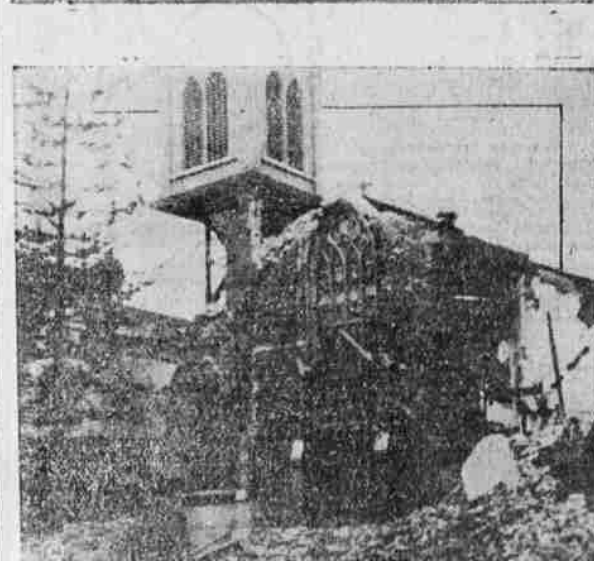
Upper—Once this building covered a whole block in Santa Barbara. Today it is a demolished structure, shaken to the ground by the earthquake last Monday. Center—This photograph shows how the Catholic church, standing alongside of the Knights of Pishias hall, was ruined. Lower—Another view of the Catholic church as it was wrecked.
