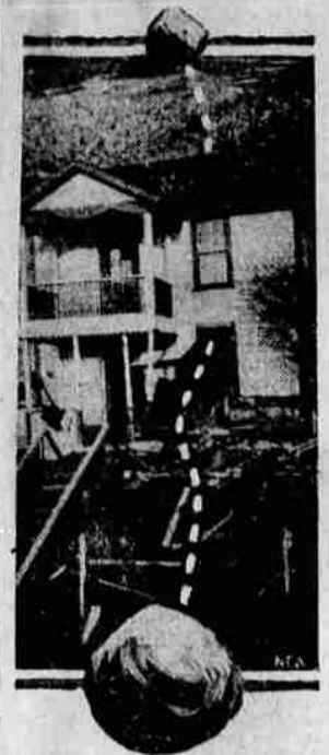
He built his house at the bottom of a hill; and he didn't build it strong enough to withstand attacks of rolling stones. Now you see what happened when a six-ton boulder set out to roll, and rolled right through the house of Steve Masters, Klamath Falls, Ore. The baby cried when his crib was upset.
