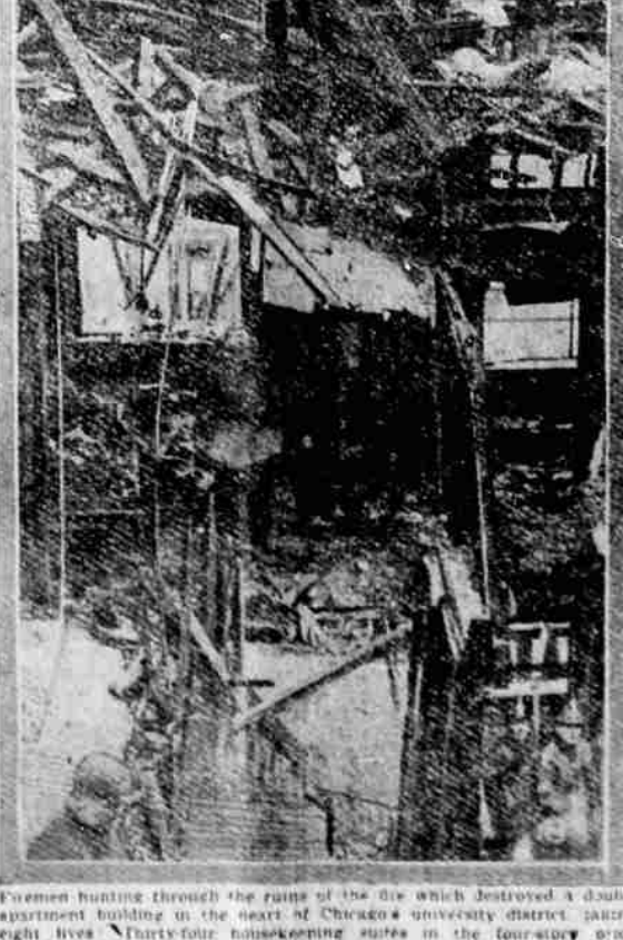
Where Eight Met Death Foremen hunting through the ruins of the fire which destroyed a double apartment building in the heart of Chicago's university district, taking eight lives. Thirty-four housekeeping suites in the four-story brick structure were reduced to ashes.
