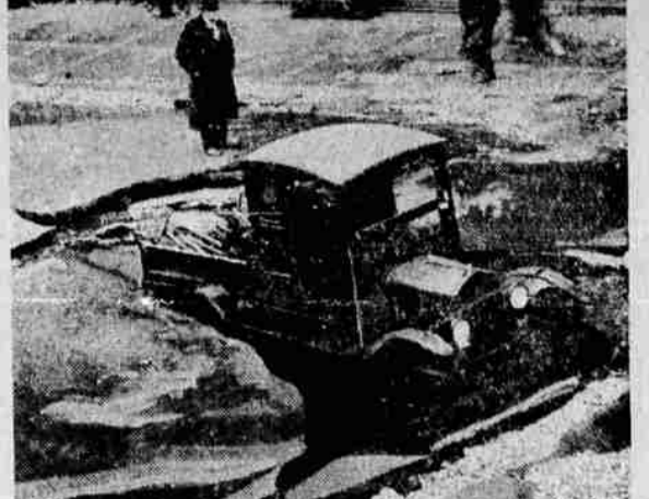
Looks like an earthquake. But it isn't. It's part of the havoc wrought by the bursting of a 36-inch water main in downtown Cincinnati. Cellars were flooded 10 blocks away. The automobile in the hole is a water works service truck. Street lights were out of commission and the driver, unable to see distinctly, drove into the hole. Six men narrowly escaped drowning.
