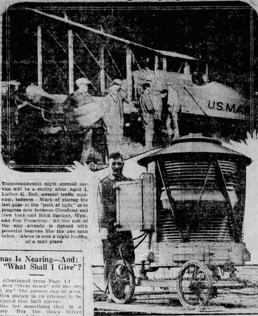
Transcontinental night, airmail service will be a reality after April 1. Luther K. Ball, airmail traffic manager, believes. Work of closing the last gaps in the "path of light" is in progress now between Cleveland and New York and Rock Springs, Wyo., and San Francisco. All the rest of the way already is lighted with powerful beacons like the one seen below. Above is seen a night landing of a mail plane.
