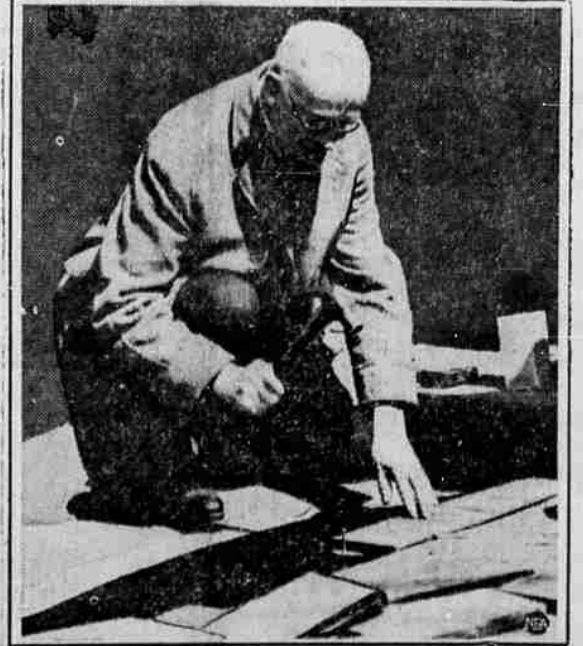
Rubber paving blocks, made from old auto tires, are being tried out in Boston streets. They are said to take the noise out of traffic and to wear better than many of our concrete blocks. John A. Houck, a Boston city official, is shown using the first blocks.
