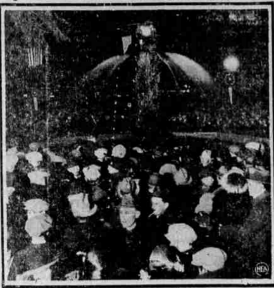
When President Coolidge touched a button in Washington the other day, this fountain of crystal water, connected with the new $2,700,000 filtration plant in Sacramento, Cal., was turned on and leaped in the sunshine. The occasion marked formal opening of the plant, and likewise ended a 40-year struggle on the city's part to obtain a clear water supply.
