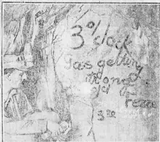
A few chalk marks on a wall of stone tell the tragedy of the 47 miners whose bodies were found entombed in the Arconaut mine at Jackson, Cal. While their fellows were working feverishly to dig through the rocks their men tried to keep a report of their suffering. These marks will stand as their monument.
