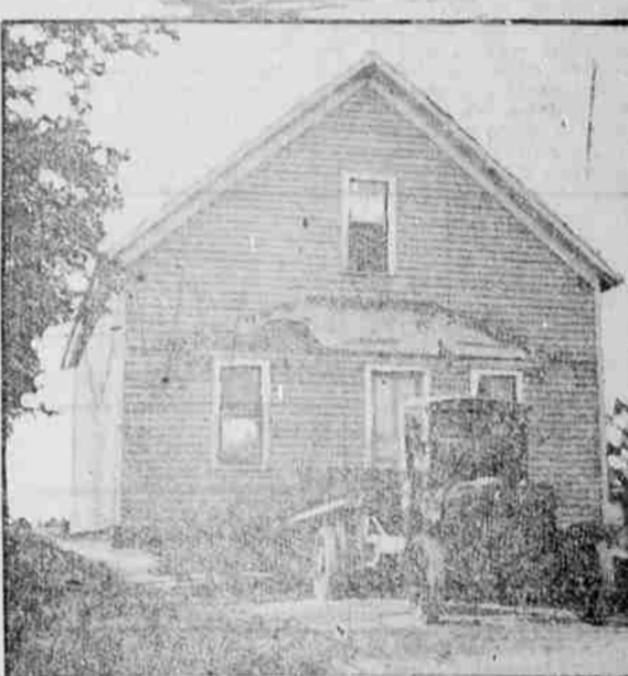
MOVING A TOWN. Now that the lumber has all been cut around Jennings, Mich., there's no excuse for the town. So all the buildings are being put on motor trucks and moved to other locations.
