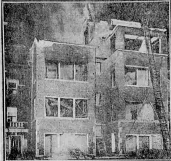
This new $500,000 "Lands award" apartment house on Sheridan road, Chicago, suffered $250,000 damage by fire after labor leaders had been jailed on murder charges.
