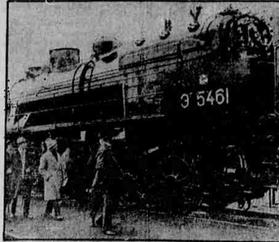
One of the new locomotives manufactured at the Essen Works for the Russian Soviet government. It's a wood burner. Notice the Soviet emblem above the engine number.
