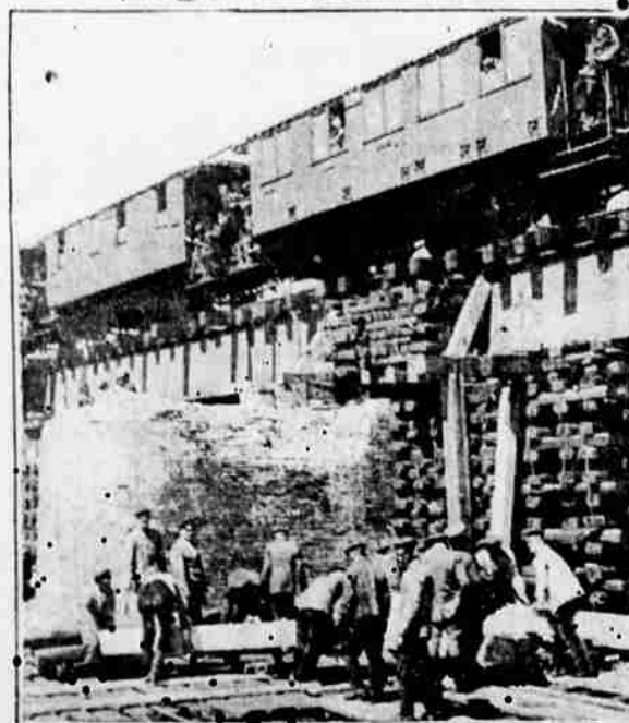
That there was real war in Upper Silesia between the Germans and Polish insurgents is shown by the picture. The Germans had to rebuild the railway bridge near Opava with logs after they had forced the
