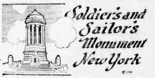
This memorial, erected on Riverside Drive, N. Y., to the memory of American Patriots, is Corinthian in its architectural tendencies, and is an excellent example of modern workmanship.
