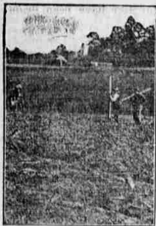
Using a Level to Lay Off a Drainage System.
