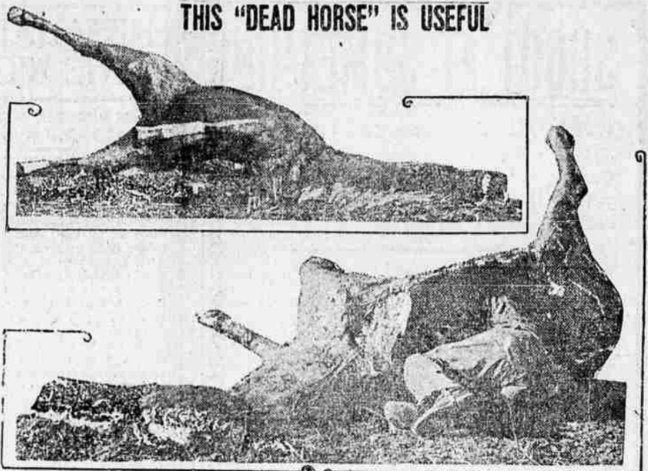
Two views of a "dead horse" that is most useful in war. The top view is how it appears to the enemy. But below it's real purpose as a listening post for American engineers is revealed. Of course, it isn't a horse at all but a fake made by U. S. army camouleurs.
