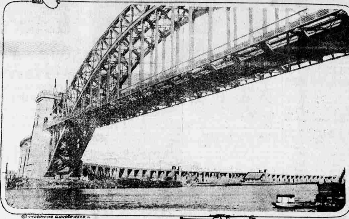
Holt Gate bridge, the largest and heaviest steel arch railroad span ever built, is nearly ready for use. The bridge connects Long Island and New York and carries four tracks. The steel span is 1017 feet long. Forty million pounds of steel were used in the massive span and 160,000 pounds in the immediate approaches. The winding steel and concrete approach is nearly a mile long.
