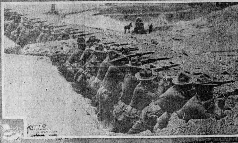
IN TRENCHES AT CASAS GRANDES
