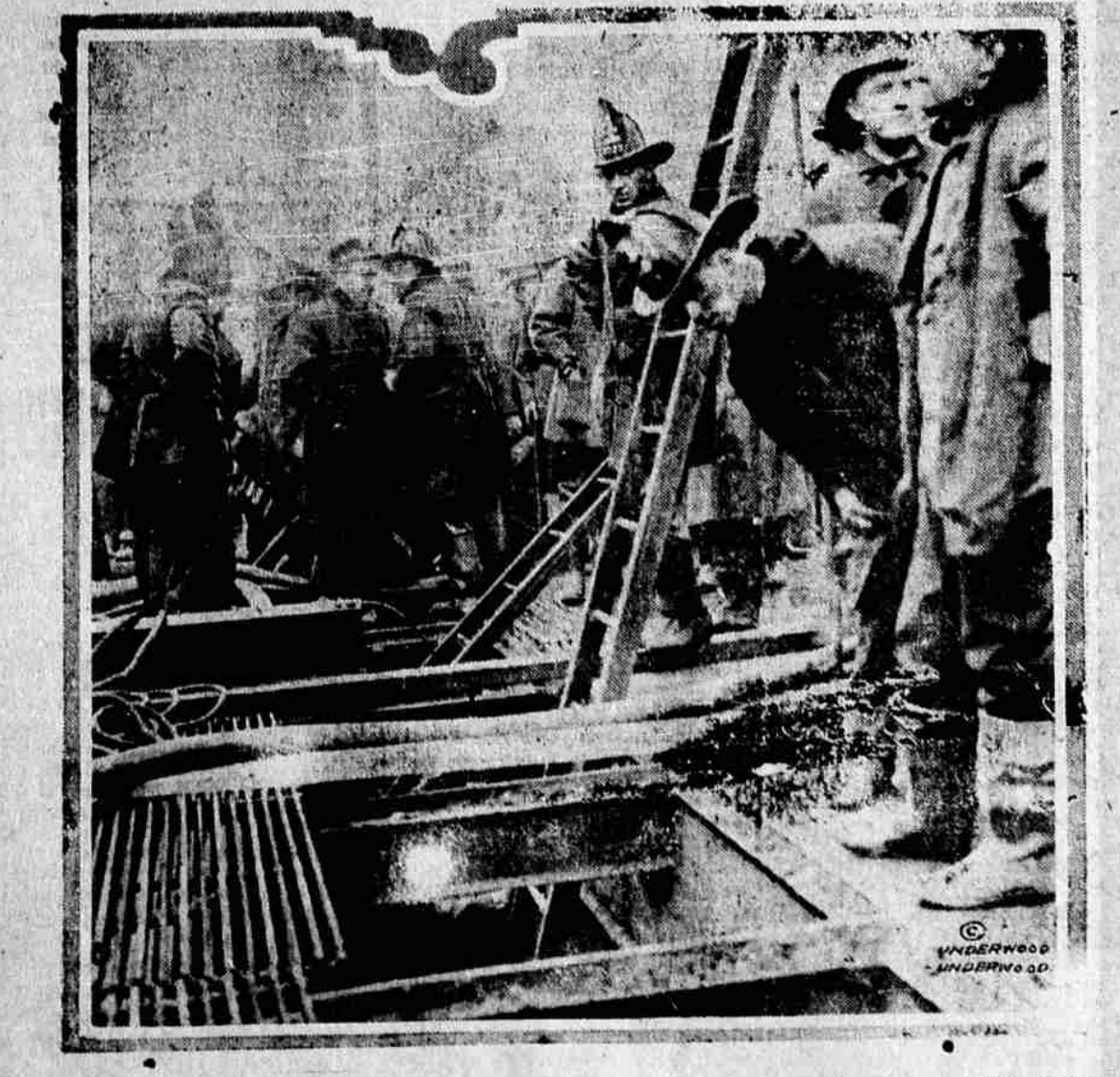
More than 170 persons, most of them half suffocated with smoke and some of them in a dangerous condition, were dragged from this hole near the heart of the busiest section of the city, when fire spread through New York's great underground tunnel a few days ago.
