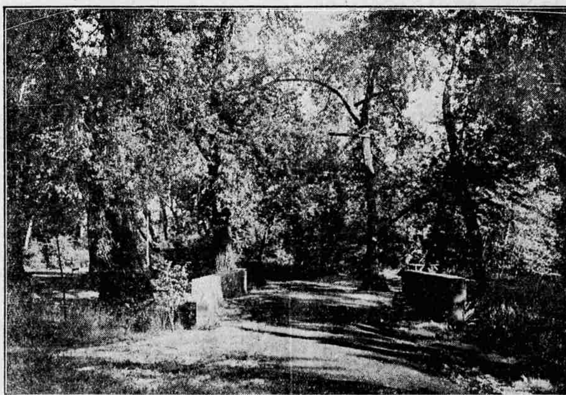
The substantial, attractive cement bridges spanning lagoons at Riverside park are admitted to be big factors in developing that tone of symmetry so conspicuous in every phase of Riverside architecture. The photographer here caught a near view of one of several similar bridges, and in the background looms the playgrounds for children. The majesty of the forest is not lost sight of in Riverside park, as witness this scene
